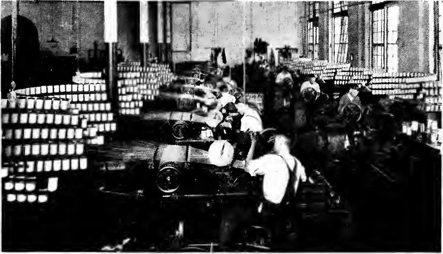
**E**ACH great lace machine requires approximately 4,000 bobbins. This photograph shows the operators winding bobbins, all of which must hold the yarn with uniform tension in the machine.
