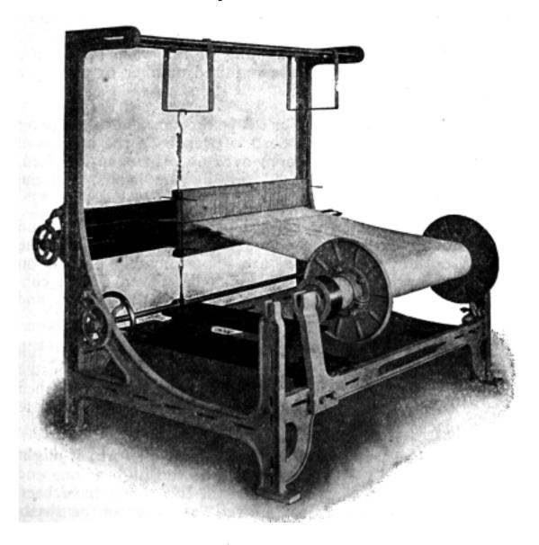
Fig. 20. Hattersley's Looming and Twisting Frame.
