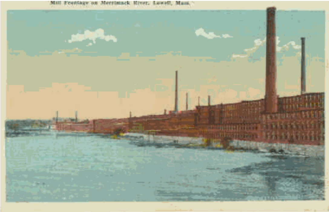
Mill Frontage on Merrimack River, Lowell, Mass.
