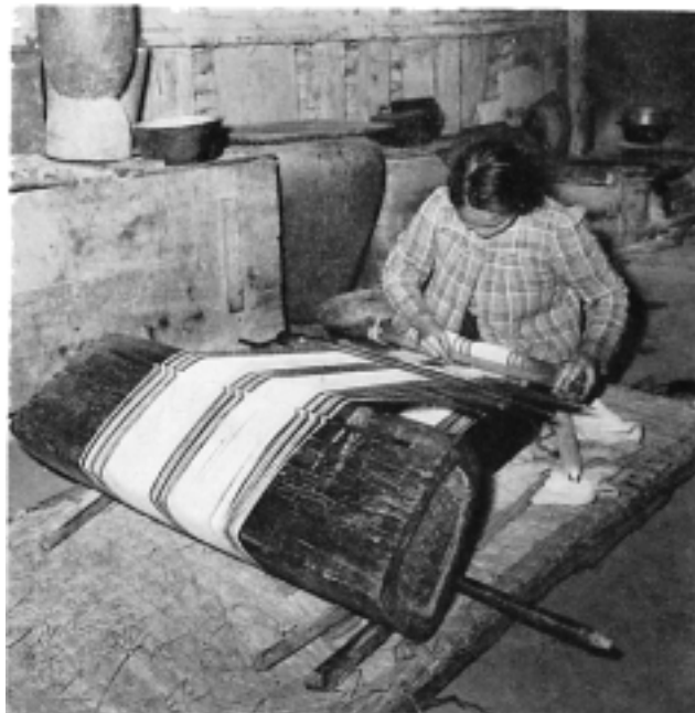
PLATE IV ATAYAL TYPE OF LOOM SHOWING END- LESS BELT OF WARP TIED TOGETHER.
