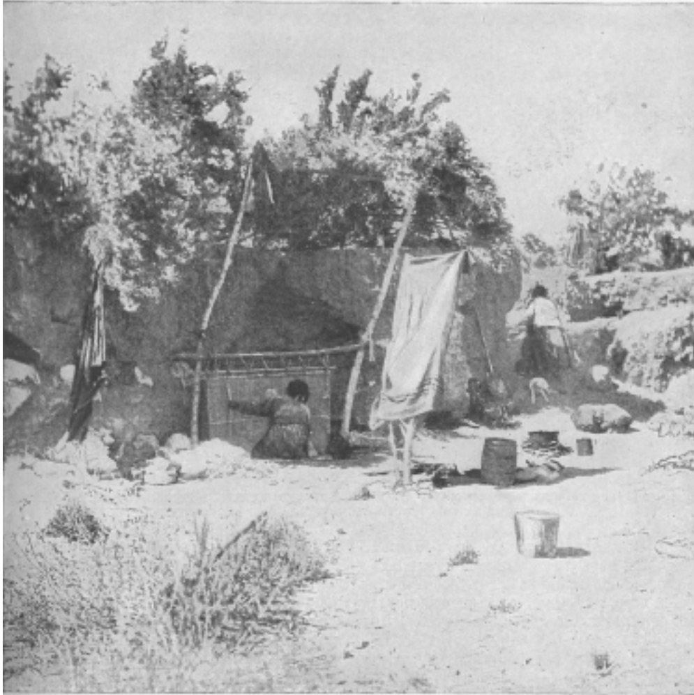
"THE HOGAN, OR HOUSE, GENERALLY CONSISTS OF A FEW TREES DRIVEN INTO THE GROUND TO FORM A SEMI-CIRCLE. THE TOP IS COVERED WITH BRUSH OR A BLANKET, BUT OFTEN . . . AN ARROYO-BENCH . . . FORMS THE BACK PART OF THE HOUSE."
