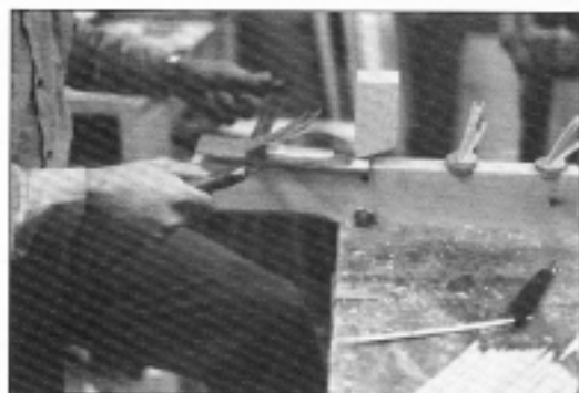
Left, harnesses fabricated from a bar on the top and a bar on the bottom and string heddles are not unlike those of present day Swedish looms.
